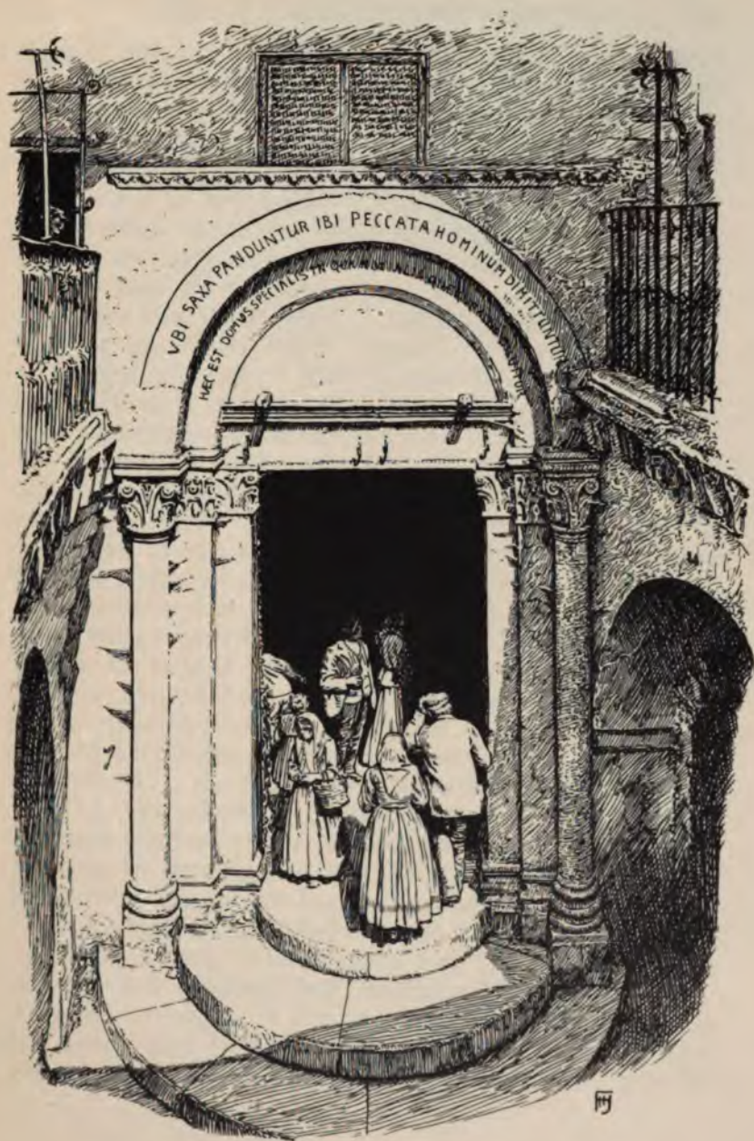
ENTRANCE TO THE GROTTA, MONTE SANT' ANGELO
